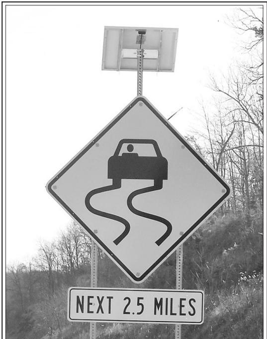
In an effort to reduce crashes on our roadways, the Kentucky Transportation Cabinet has installed a new safety device on two sections of I-75 in Laurel and Rockcastle Counties. Flashing LED enhanced signs have been erected warning motorists of "Slippery When Wet" pavement conditions.
