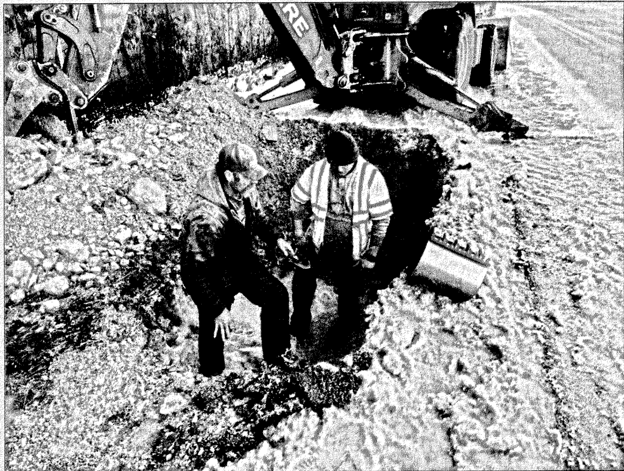
Shown above, Lloyd Prewit and Keaton McClure work on one of many frozen water lines Monday. This location, near Pizza Hut, is one of many that forces workers to stand in water and mud in below freezing temperatures to repair such leaks. A boil water advisory was issued Monday for the Burr area, Big Cave Road and all side roads off of Big Cave Road but is expected to be lifted by mid-week.
